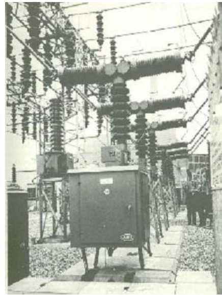
132kV Live Tank Vacuum Circuit Breaker
