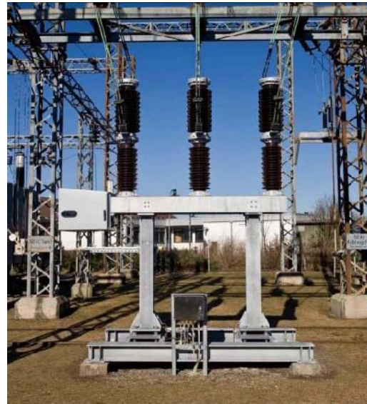
72.5kV Live Tank Vacuum Circuit Breaker
