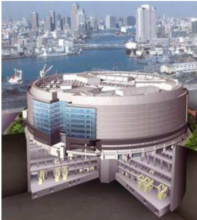
550 kV Shin-Toyosu underground substation [118]
